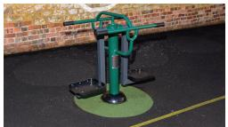
Referred to as soft surface, rubber chipping, rubber tarmac and many other names, wetpour is quite simply rubber chips of a certain size mixed together with a specialist glue and laid flat on the ground to create a safety surface.
